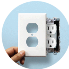
STEP 1 Shut off the power and remove the wall plate from the outlet
